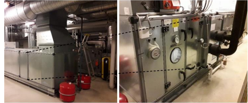
Exhaust air ventilation and the additional heat exchanger (HE7) (Korpela 2021, Xamk)
